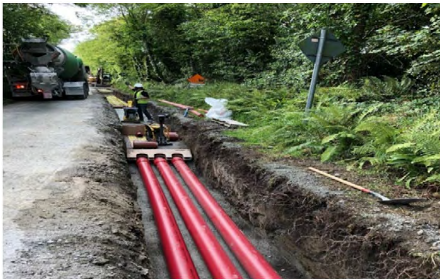
Figure 3-6 Typical HV Cable Duct Installation in Public Road 7
