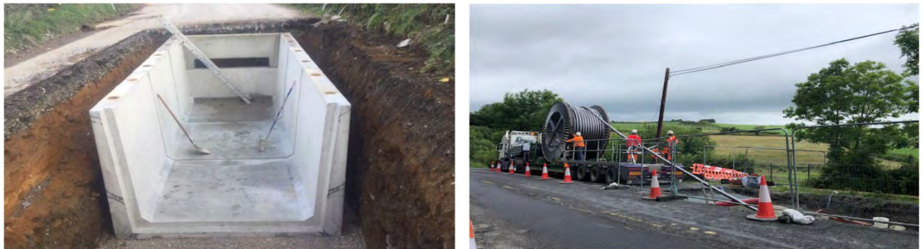
Figure 3-8 Typical HV Joint Bay and Cable Installation 8
