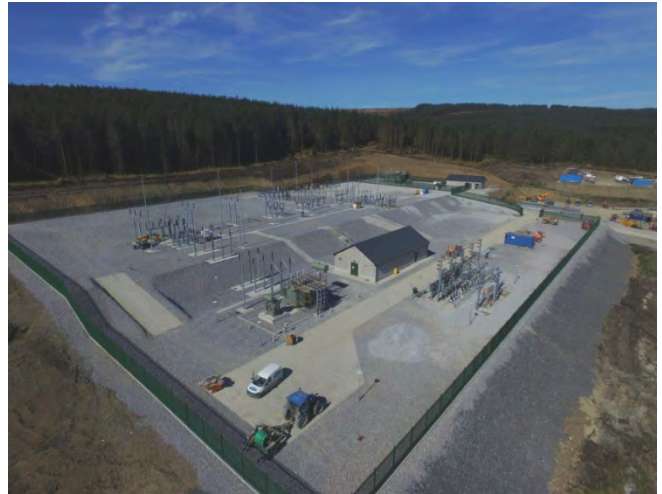
Figure 3-10 Example Gas Insulated Switchgear Substation Building and AIS Substation Compound 1011
