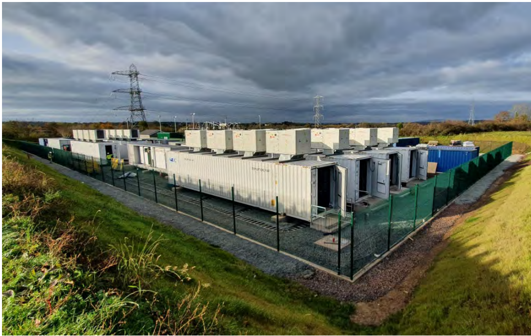
Figure 3-11 Typical Battery Energy Storage System (BESS) Compound 12
